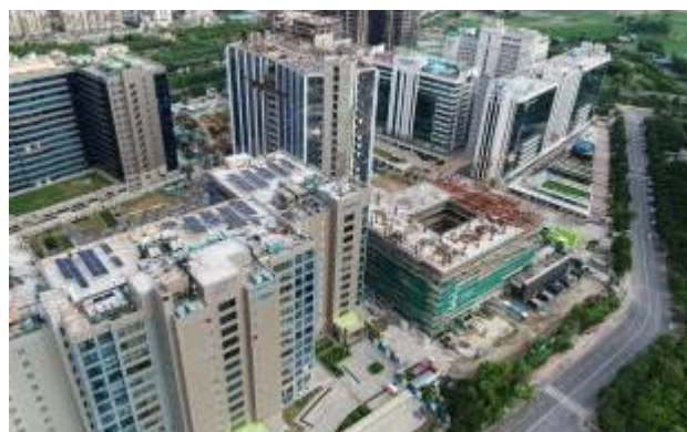
Tower 11 A (as of September 2020)
